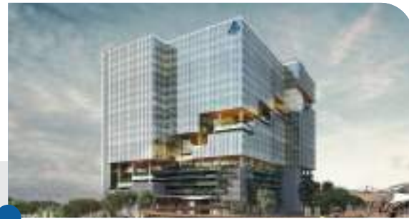
Building 8, Mindspace Madhapur
