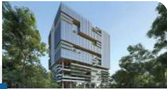
Building 1, Mindspace Madhapur
