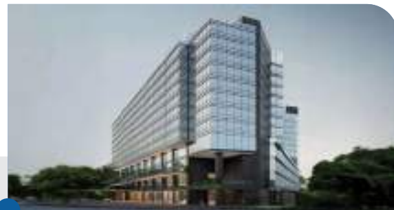
Building 18, Mindspace Madhapur
