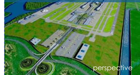
Navi Mumbai International Airport
