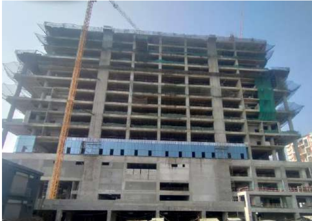
Commerzone Kharadi, Pune Building 4 (~1.0 msf)
