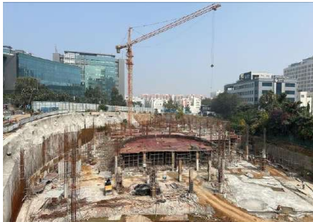
Mindspace Madhapur, Hyderabad Experience Center (~0.13 msf)
