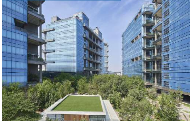
Gera Commerzone Kharadi Pune | 3.0 msf (1)
